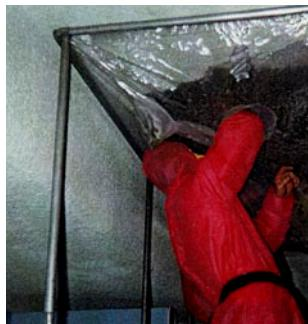
**Figure 7.18** A glovebag designed for the removal of sprayed asbestos coatings. Note the gloveports, waste chute and vacuum nozzle used for cleaning and providing slight negative pressure
