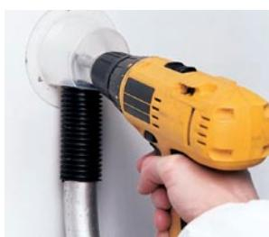
**Figure 7.7** Textured coating being drilled through paste
