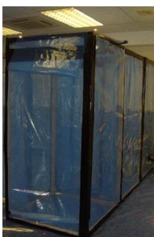
security sheet on the outside) which is used to cover over the entrance at the end of the shift. It should be taped back onto the roof area when the airlock is being used.
