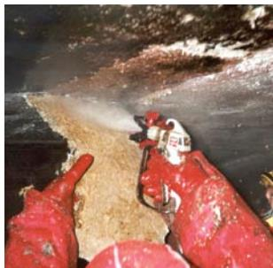
***Whichever approach is taken, every effort should be made to ensure that the lagging is as uniformly wetted as possible before stripping.
